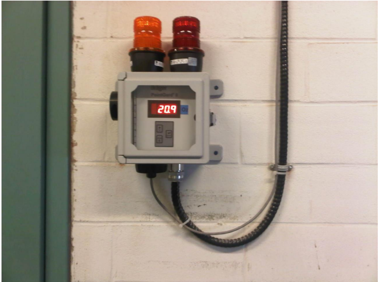
Figure 5. The LNDF's oxygen sensor. The oxygen level value display is located just outside the LNDF.
